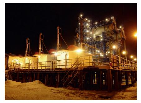
Low pressure booster compressor station on the basis of Energroject units pumps low-pressure associated gas at the Varandey field of LUKOIL-Komi
